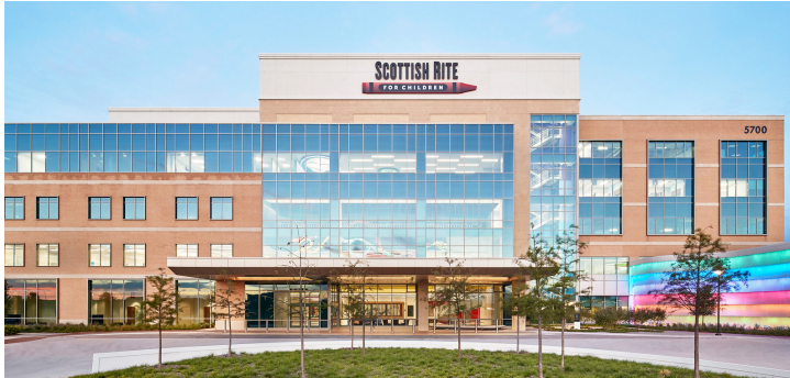
At the northeast corner of Lebanon Road and the Dallas North Tollway.
